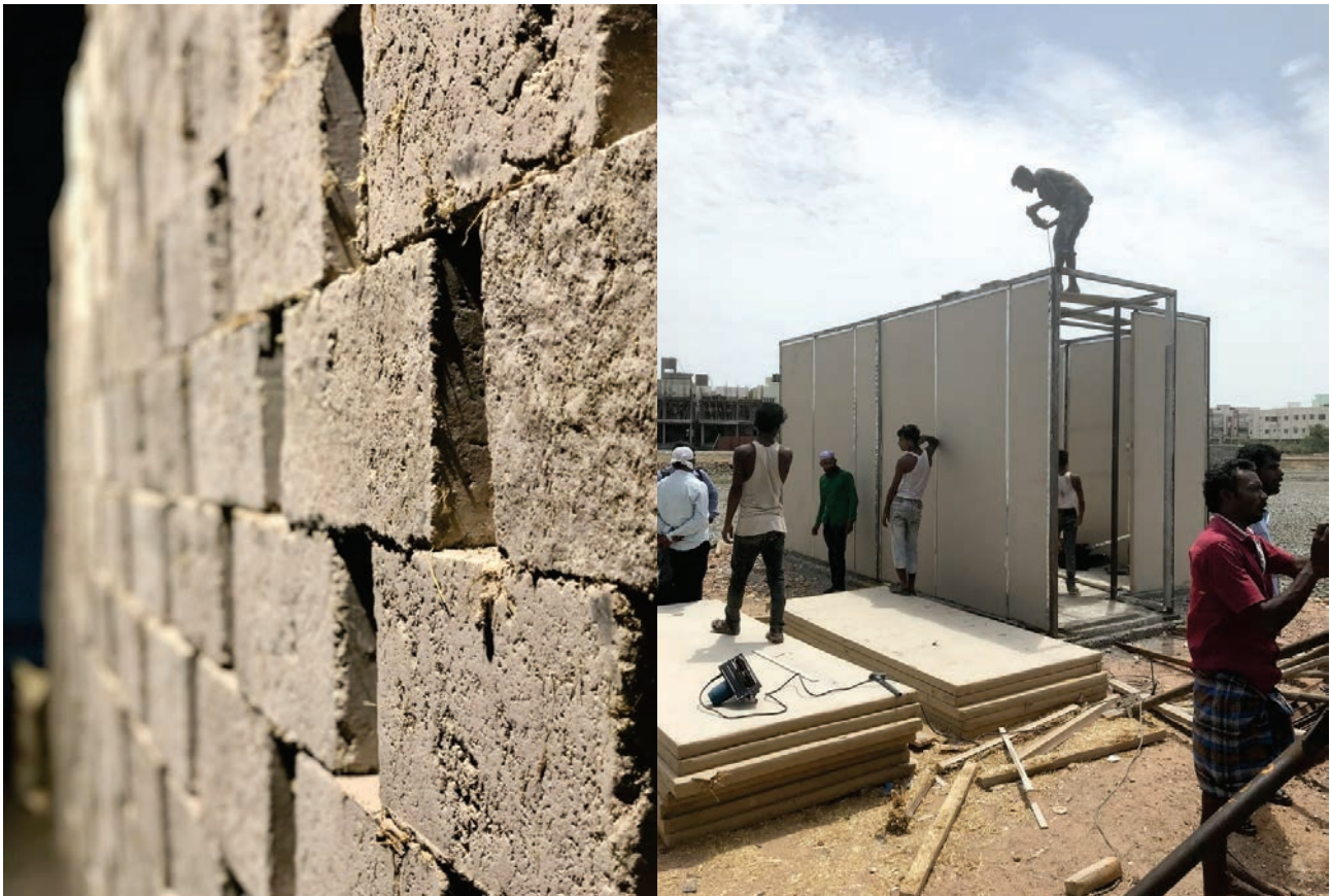
Figure 12. Agrocrete blocks and strawboard panels from Strawture Eco
