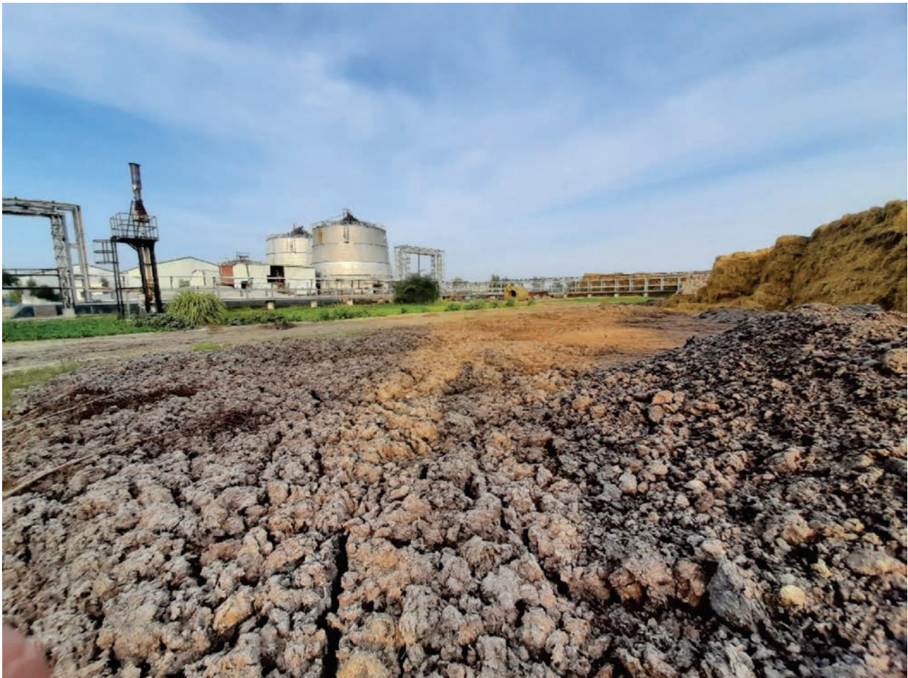
Figure 11. Bio-fertiliser offtake is crucial for viability of Bio-CNG model: Sampurn Agri Venture's Bio-CNG plant in Fazilka, Punjab with green manure from plant being cured in open as seen in the foreground
