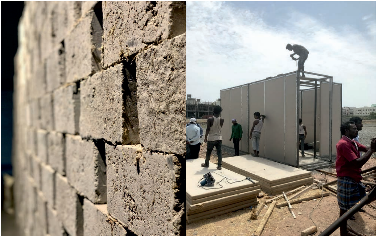
Figure 12. Agrocrete blocks and strawboard panels from Strawture Eco
