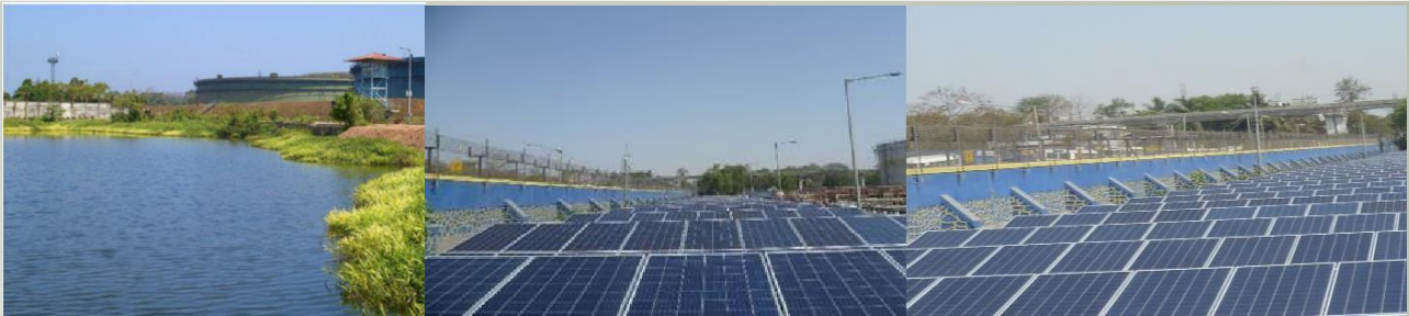
(L to R) Water harvested in Kochi refinery and solar power plants at different locations
