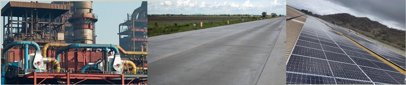
(L to R) Blast furnace gas utilisation; Steel slag road in Hazira, Surat; Solar panel installation
